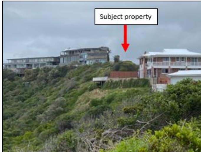
Figure 8: A photograph of the subject property and the surrounding neighbours.
